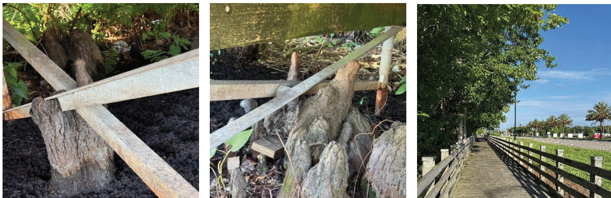
Photo 15: Tree roots impacting steel braces (left, center) and overgrown vegetation along boardwalk.
