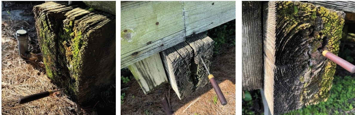
Photo 12: Rotted beam ends
