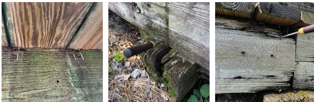
Photo 13: Joists with deck fasteners improperly installed along edge, rot at bearing, rot at top edge (from left to right)
