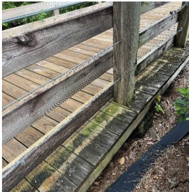
Photo 5: Pressure washed deck planks on west end of boardwalk
