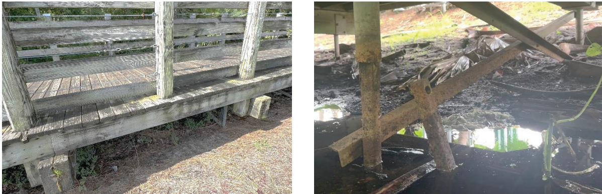
Photo 1: Galvanized steel helical piles in dry land vs. wetland (from left to right)
