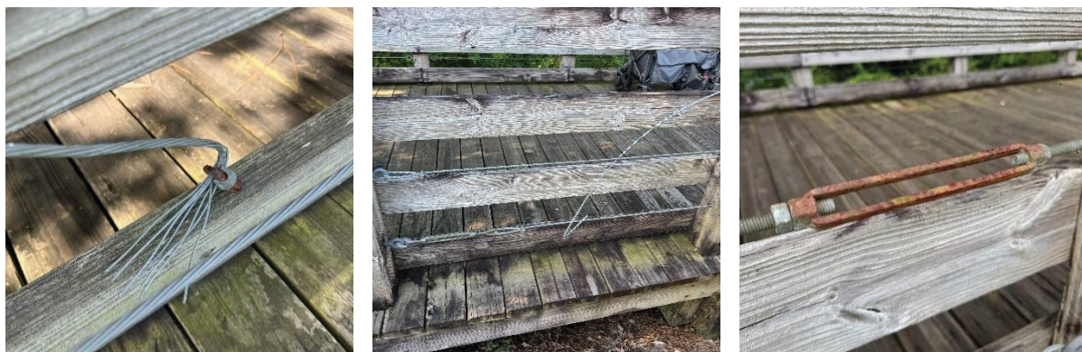
Photo 6: Loose cable rails and connectors with surface rust
