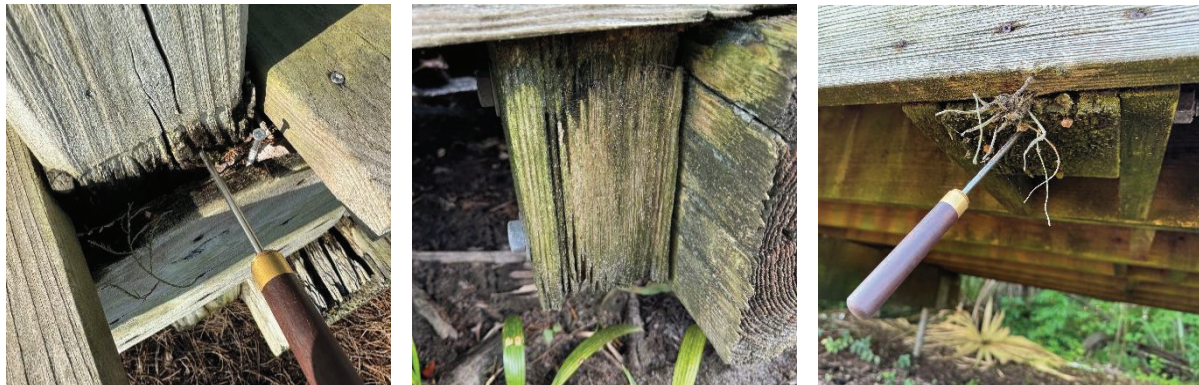
Photo 8: Guardrail post rot at rim joist (left) and at the end grain (center, right)
