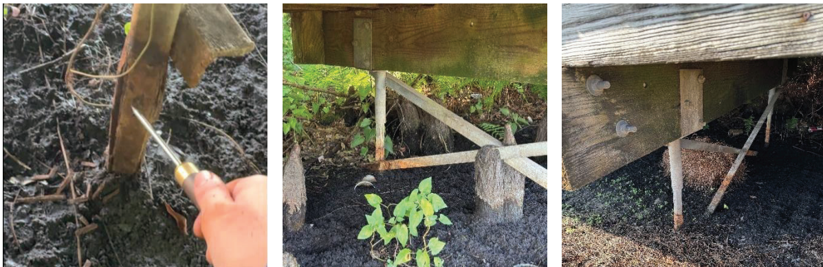
Photo 11: Steel angle brace and helical pile with corrosion
