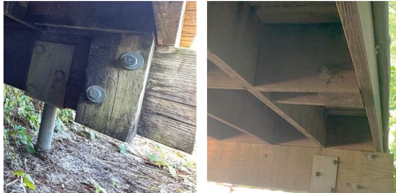
Photo 7: Rigid guardrail construction, bolted to beam (left) or bolted to vertical blocking (right)
