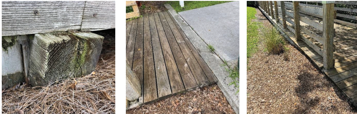
Photo 9: Locations of rotted wood framing in contact with soil
