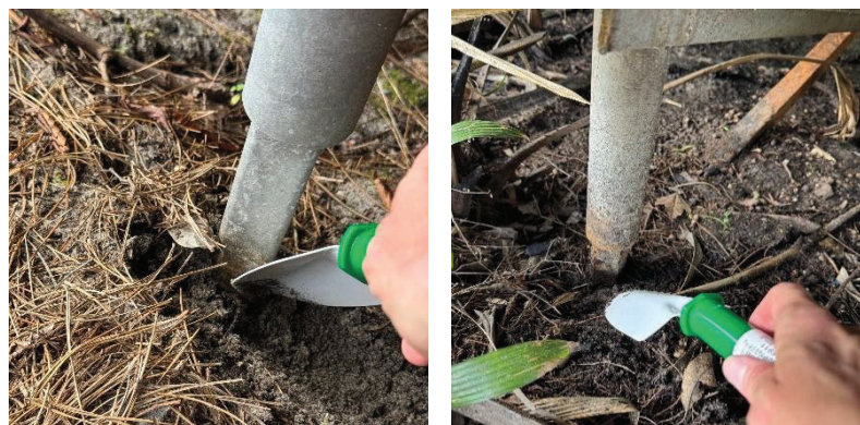
Photo 4: Excavation of steel helical piles and braces using a hand trowel
